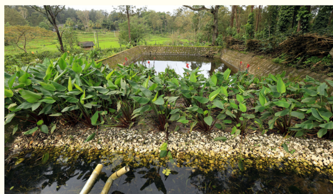
Constructed Wetland Treatment System to treat coffee pulping effluent | Source: Firefly Life Sciences
